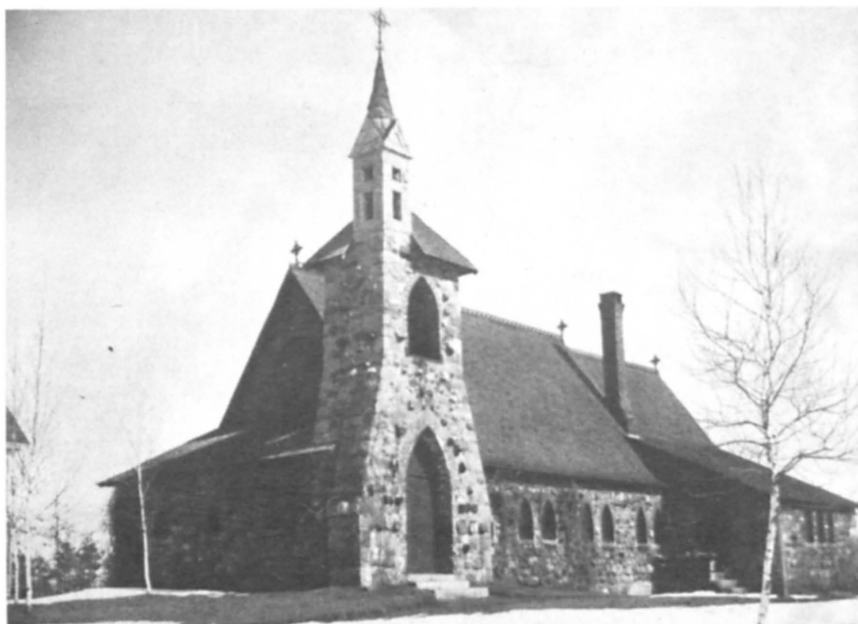
Christ Episcopal Church, School Street, about 1885. Elmer Videtto not only built all of the masonry, but brought all of the stones to the site. The church was designed by the architectural firm of Earl & Fuller.
