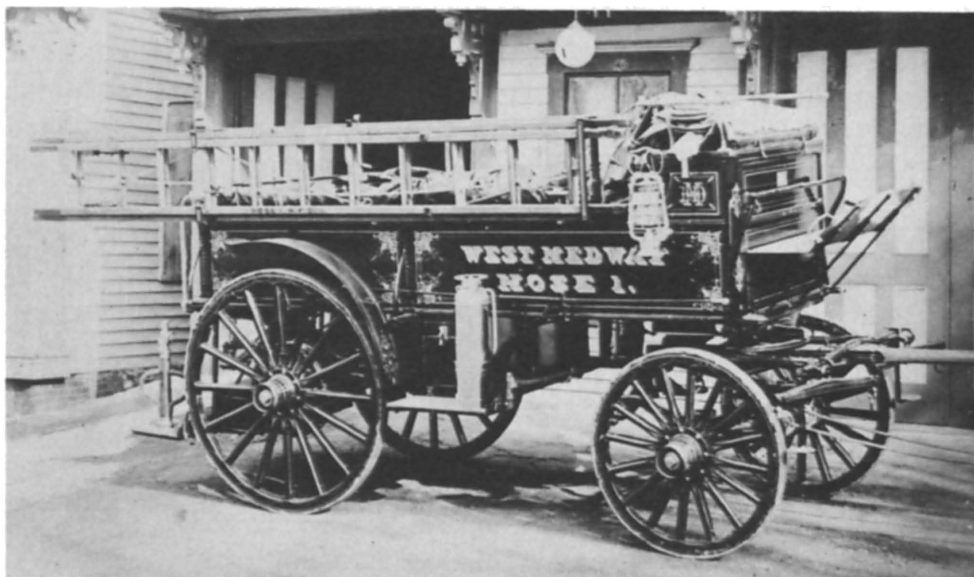
West Medway Ladder Combination at the Torrent Engine House 1911
