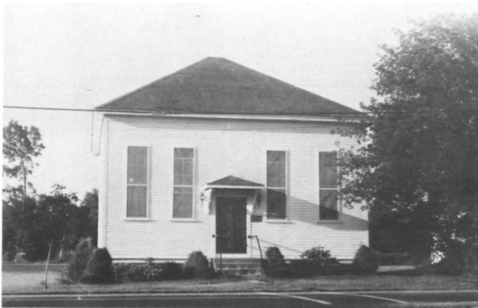
Congregation Agudath Achim Synagogue, at Walker and Village Streets, built 1919.
