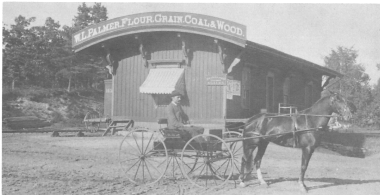
Walter L. Palmer in front of his place of business, 1895. The building was the original New York & New England RR depot at Medway. It was of the same architectural style as the first depots at West Medway and at Walker Street on the Medway Branch RR.
