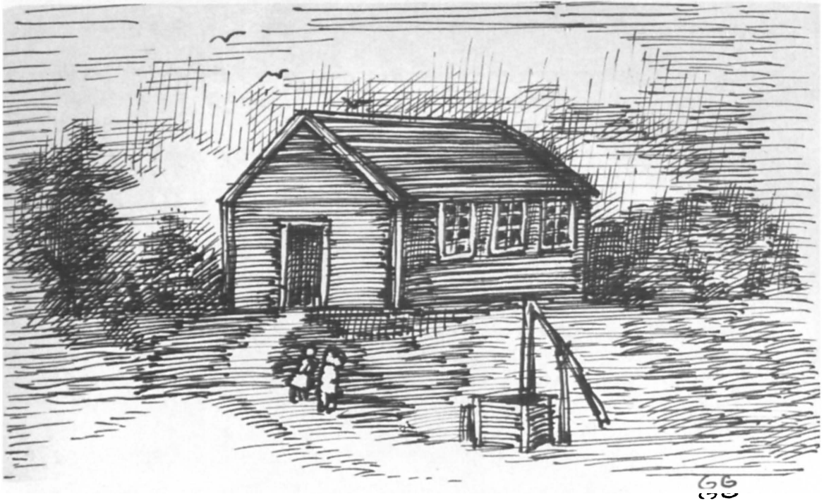
The Drybridge School - Typical of Medway's early one-room schools.
